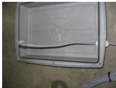
Figure 6. Secure connector to the cable
