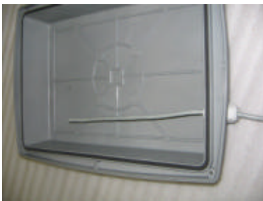
Figure 5. Insert cable through gland
